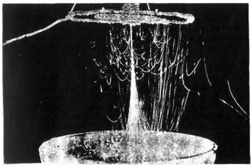
Motion of Charged Water Particles around the Spiral Charge Collector Photo from the Swedish Biotechnical Research Institute
